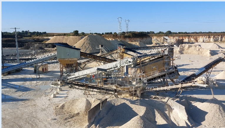
Installation de criblage
